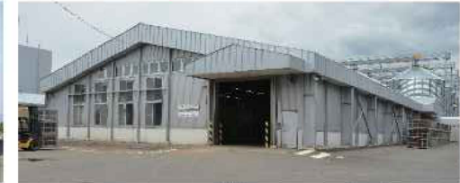
4 Chinese yam washing and sorting facility: Built in 1991/Equipment update: 2015
