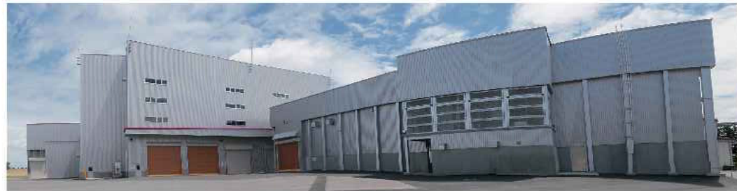
6 Beans storage and preparation facility, Beans cold storage facility/60,000bags: Built in 2018
