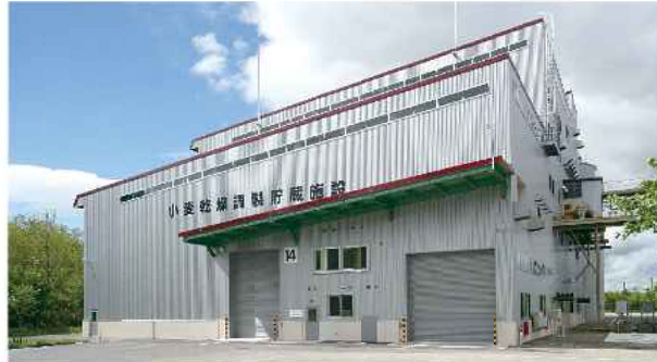
3 Wheat drying preparing and storing facility/9,000t: Built in 2008
