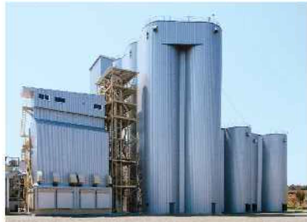
3 Wheat drying storing facility/9,000t(1,125t×8units): Built in 2011 9,000t(500t×18units): Built in 2008
