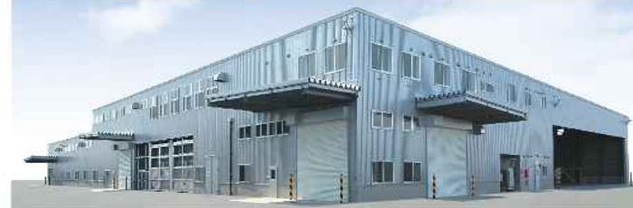
4 Carrot washing, sorting and pre-cooling: Built in 2006
